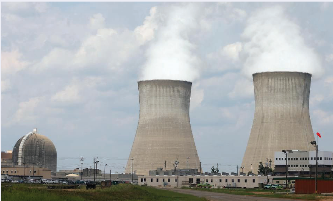
Photo of the cooling towers and nuclear reactor containment building at Plant Vogtle Nuclear Power Plant in Waynesboro, Georgia. Westinghouse Electric Co., the U.S. nuclear unit of Toshiba Corp., Japan, filed for bankruptcy protection on March 29, 2017. Source: AP Photo/John Bazemore.
